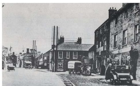
26. – ‘Ponteland’ (Main St. c.1930) In this photograph, provisions are still being delivered to the Seven Stars by horse-drawn van; the offices of the Ponteland Motor Car Co., are located in part of the former Albion Temperance Hotel; and Miss Kirkup, the chemist who occupied the rest of the ground floor, gets into her open-topped Morris.
